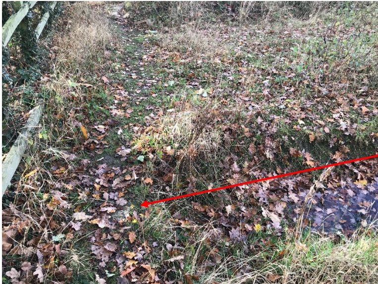
Narrow access to the side of a culverted ditch
